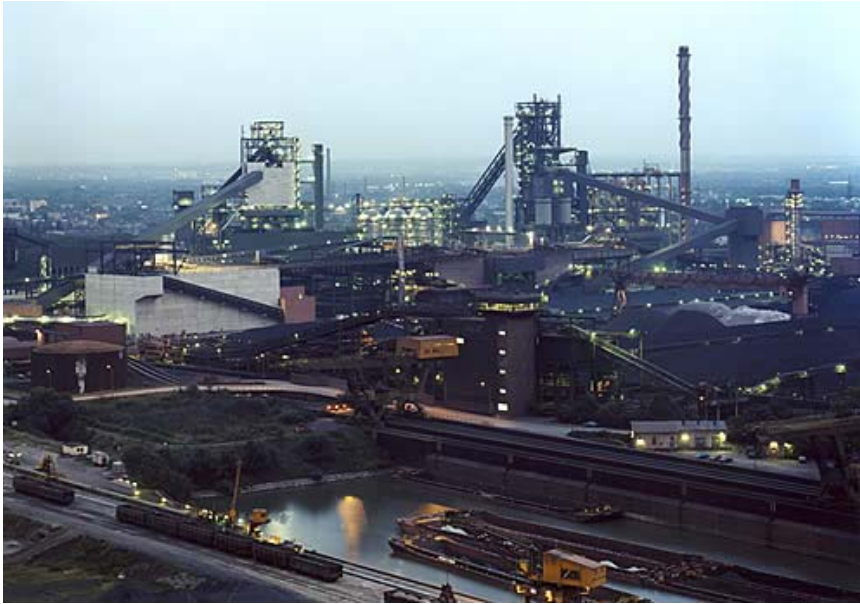
Plant TISSEN-Krupp plant, 27,000 I/O controlled by 18 operator stations
