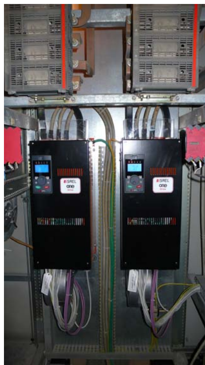
Equipment view - The old inverters replaced by the “ONE DRIVE Platform”
