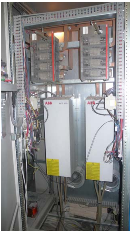
Equipment view - The old inverters replaced by the “ONE DRIVE Platform”
