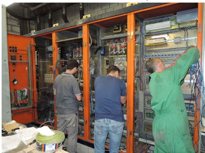
Cabinet re-use with wiring operations and REEBORN ONE
