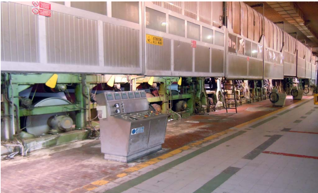
Dryer section machine 1 view - Avezzano
