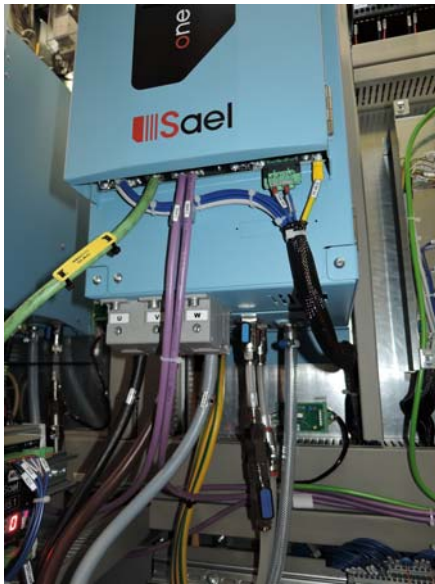
Detail of the inverters series WATER COOLING , exclusive series of “PLATFORM ONE” of SAEL
