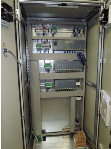
The new electrical cabinets for TURBOGAS Nuovo Pignone and the drives of the machine, PM5 Vignaletto.
