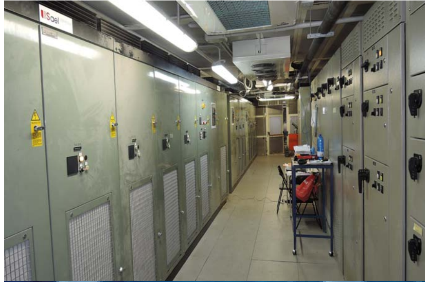
The new electrical cabinets for TURBOGAS Nuovo Pignone and the drives of the machine, PM5 Vignaletto.
