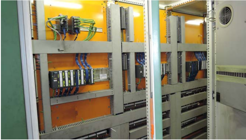
UP: PLC S7 300 used vs. the old 115U
