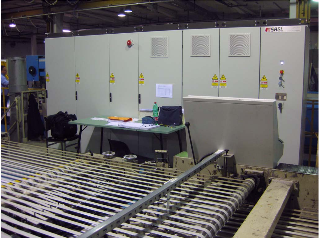
New cabinet after the complete reconstruction -step2-
