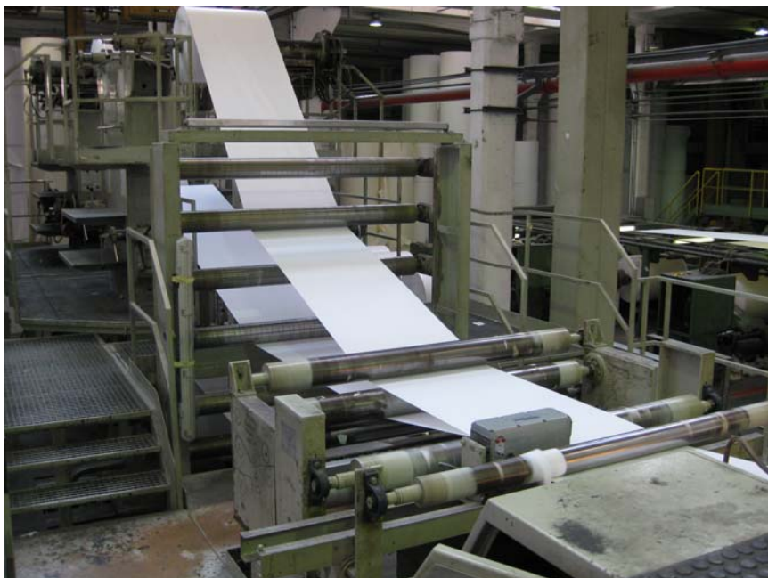
View of unwinding station of the sheeter Jagenberg
