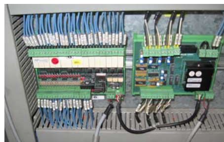
Dismantled I/O Remote boards. Valmet S5 PLC
