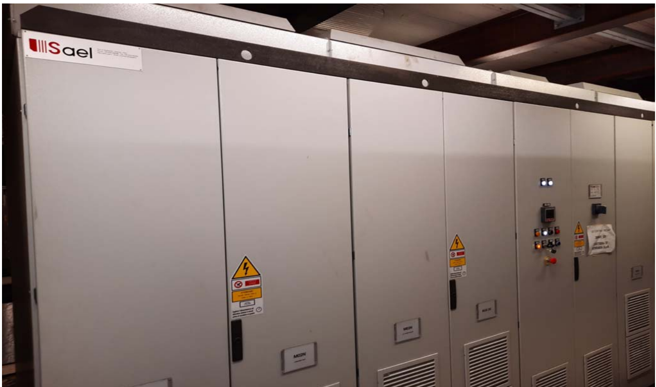
THE CONTINUOUS MACHINE ELECTRICAL CABINET, MADE IN DOUBLE END TO REDUCE THE DIMENTIONS.
