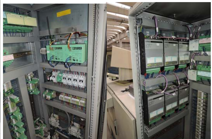
From top to bottom: Micromatik Rack, Interbus electro valves, Micromatik drives replaced and all the Interbus electronic eliminated (ET200 Siemens recycled only).
