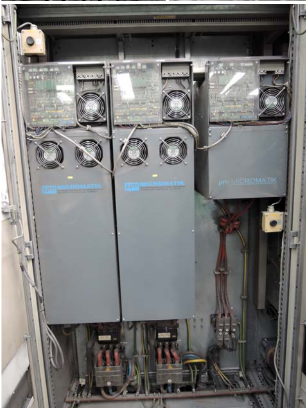
From top to bottom: Micromatik Rack, Interbus electro valves, Micromatik drives replaced and all the Interbus electronic eliminated (ET200 Siemens recycled only).
