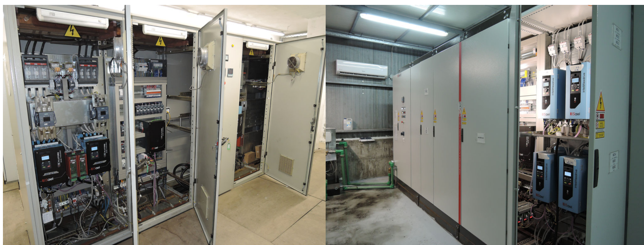
SAEL Cabinet: left the press in DC, right all the rest in AC – SAEL PLATFORM ONE DRIVE–
